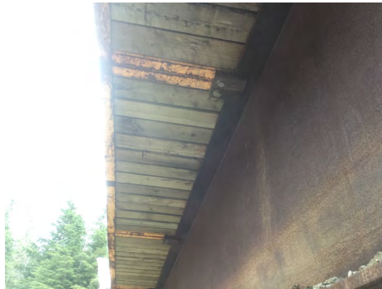
Deck clips in place and functional
