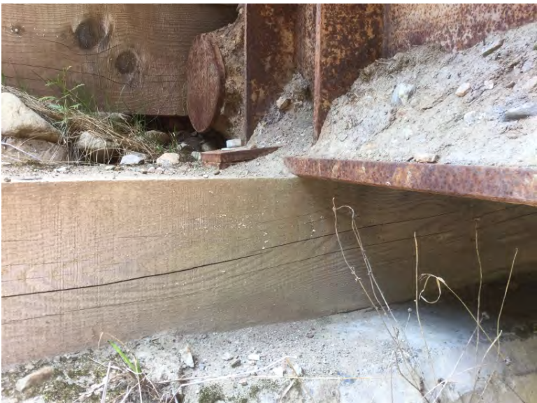
No timber sill crushing evident at right abutment
