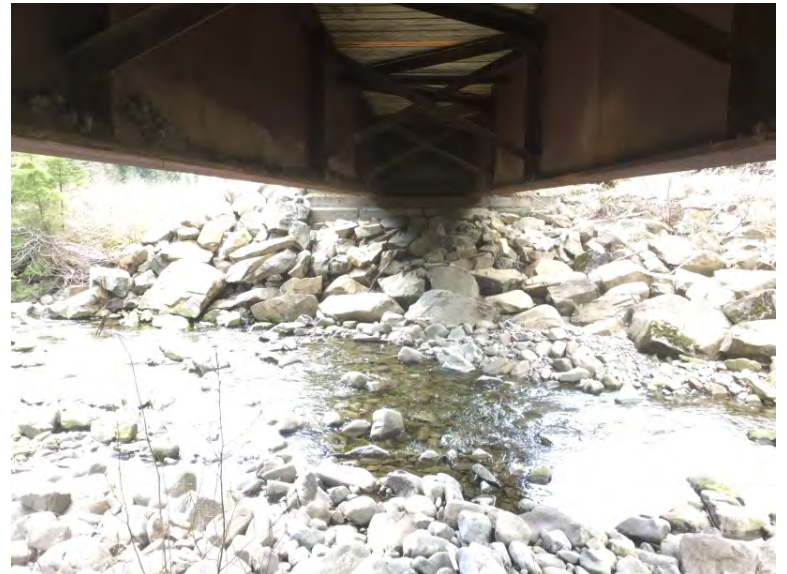
Right Bank Abutment when facing downstream
