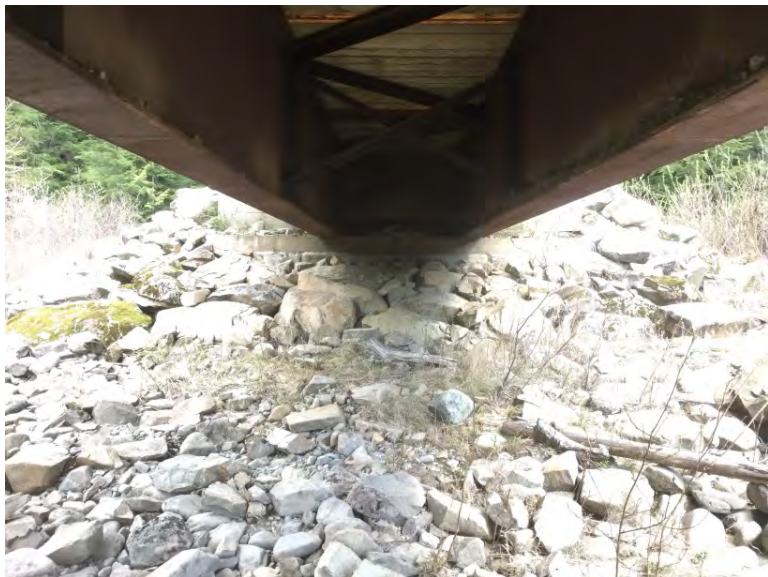
Left Bank Abutment when facing downstream
